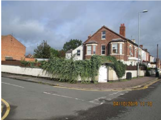
South west (side) elevation of main house
